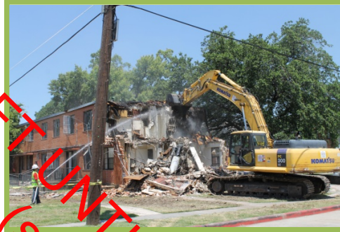
Demolition of a vacant building at Kelly Village
