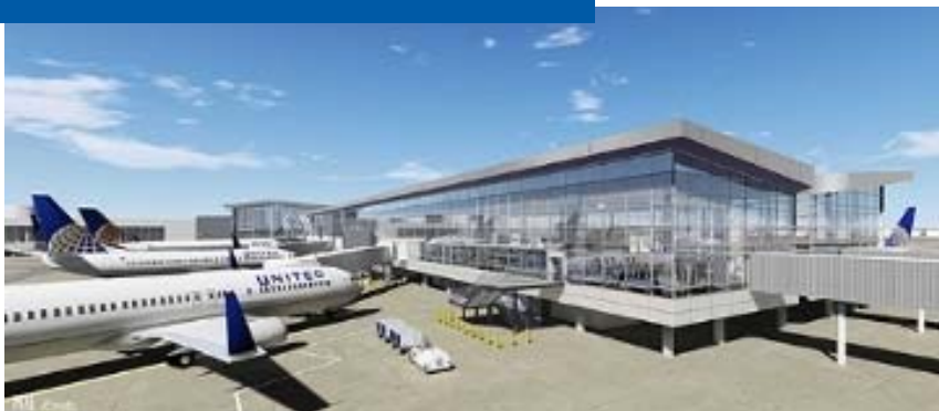
New C-North concourse
