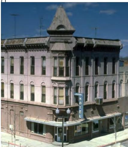
A commercial building before rehabilitation
