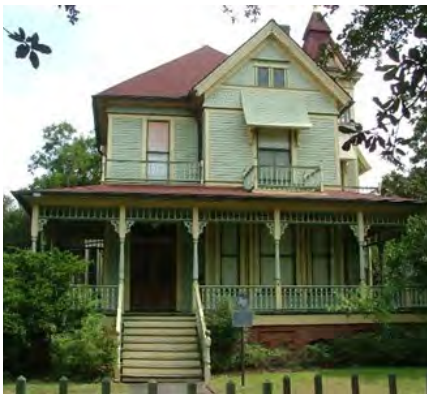
Awnings are still present on the Milroy House today.
