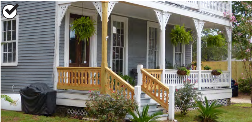
Replacement porch elements (unpainted) match the original components.
