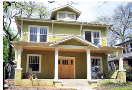
Reconstruction of the porch on a historic house: (top) before; (bottom) after
