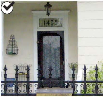
This door with a transom above is appropriate for a Victorian-era house.
