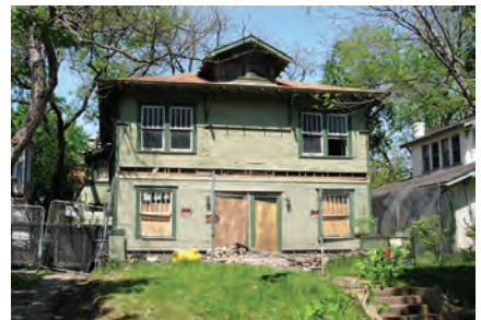
Restoration to a previous period by removal of "stone" paneling
