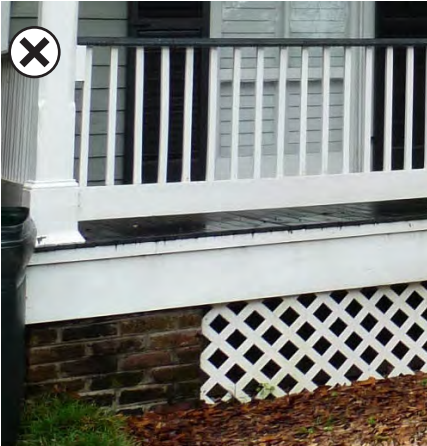
Screening panels may be installed between foundation piers. Screening panels should be framed around the lattice pieces.
