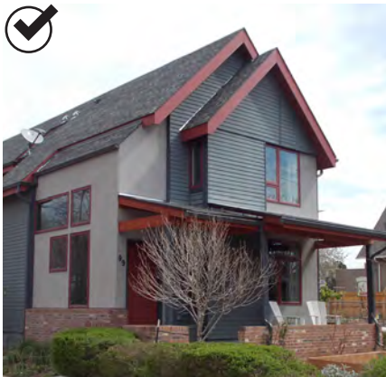
This example of new infill with contemporary design is compatible because of the mass, form and building elements such as the porch.
