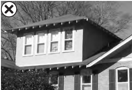
This dormer overwhelms the house and is inappropriate.
