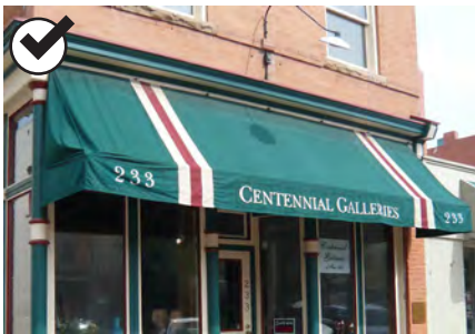
Maintain awning frames and any moving parts.
