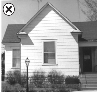
Before: A historic house with inappropriate synthetic siding
