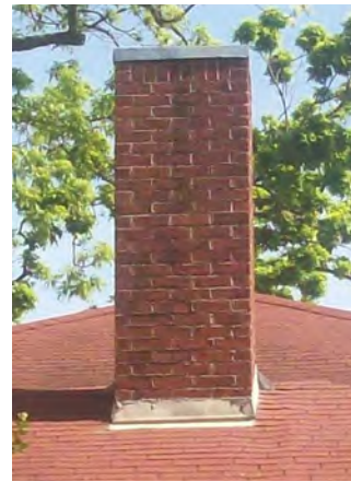
A typical brick chimney
