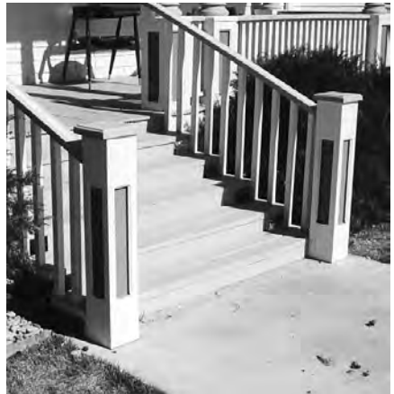
After: Handrail repaired and the post replaced in kind
