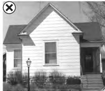
Before: A historic house with inappropriate synthetic siding
