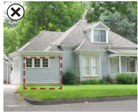
This one-story addition to the side of a historic building is subordinate in scale, but the offset wall obscures the original rear corner in a highly visible location.
