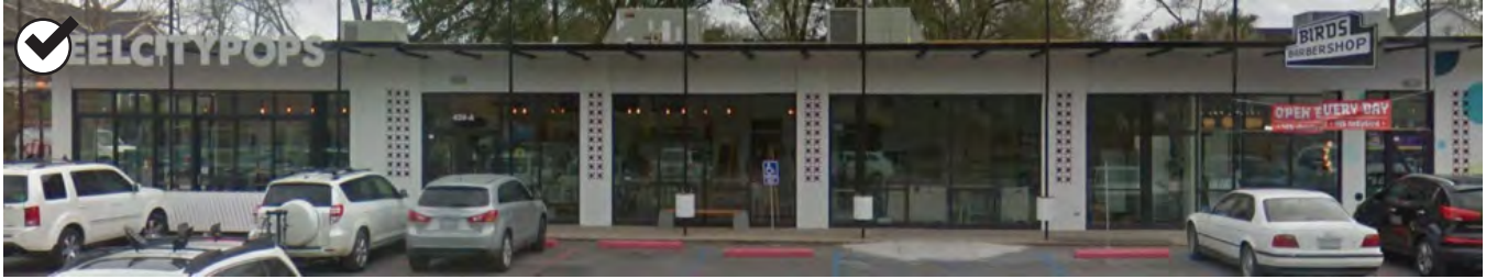
A noncontributing building with signs located within allotted storefront space, placed above entrances along the canopy
