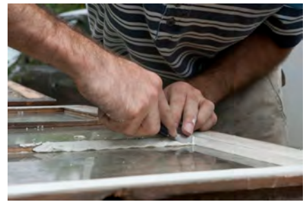
Replacing glazing putty © iStockPhoto.com/Elaine Odell
