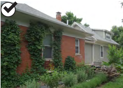
This is a compatible rear addition even though it is slightly taller than the historic building. It is compatible because it is offset, separated by a hyphen and uses compatible materials.
