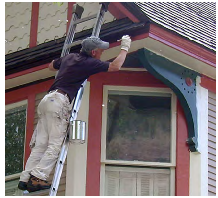
Preservation of historic materials
