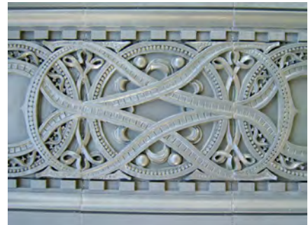
Historically, metals were used for a variety of applications, including columns, roofs, balcony railings, and other decorative features.
