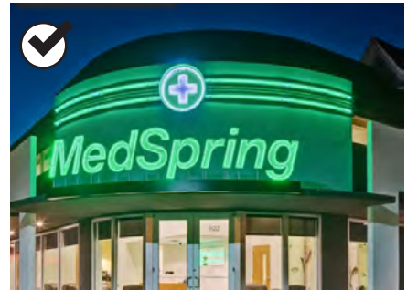
Open faced, individual letters inset with neon lighting, located above the entrances and canopy on stilts instead of against the wall face
