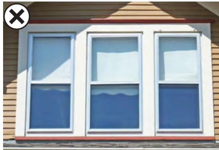
Unfinished metal windows such as these alter the character of window openings, and should not be used in highly visible locations.
